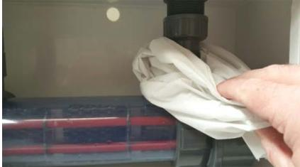
8.1.5 Loosen the union connections (a strap wrench may be used carefully to assist) and remove the union gaskets for safe keeping.
