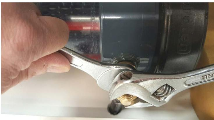
Place a 19mm spanner on the thin locking nut and an adjustable spanner on the front cable securing nut. Take care to hold the locking nut steady whilst turning the front securing nut anti-clockwise to loosen it. Repeat this procedure on the remaining terminal and remove the brass nuts and washers for safe keeping. Ease away the cable lugs from the threaded terminal bar; the cable glands
