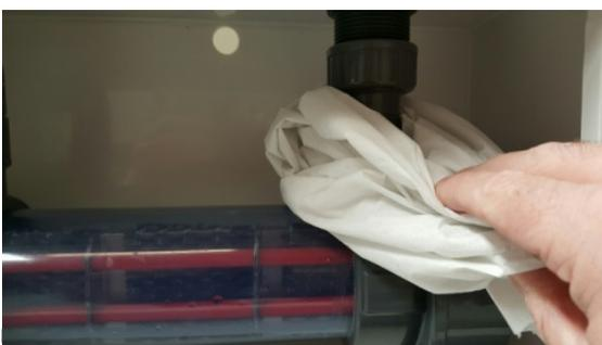
7.1.4 Loosen the union connections (a strap wrench may be used carefully to assist) and remove the union gaskets for safe keeping.
