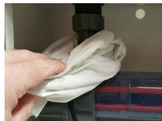
6.1.6 Slowly loosen the union connections and remove the EPDM gaskets for safekeeping.
